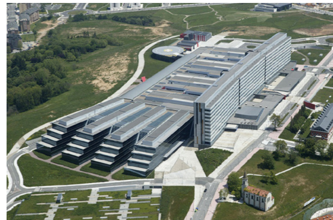
HOSPITAL UNIVERSITARIO CENTRAL DE ASTURIAS Asturias (Spain)
