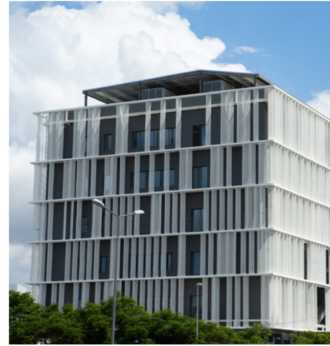
HOSPITAL CUF LOURES Loures (Portugal)
